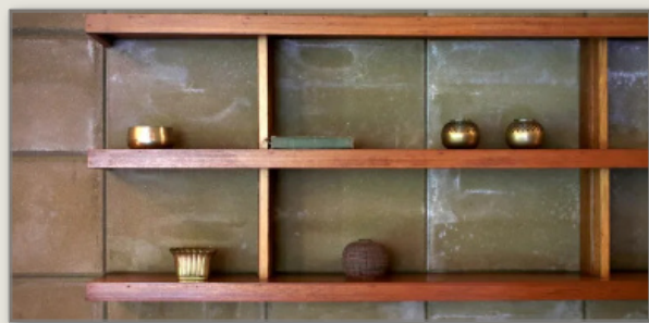
Shelves in the gallery are follow the vertical unit system of the block
